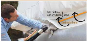
Instead of tucking the shrink wrap film under the perimeter band (like you would with a traditional recreational boat), **the shrink wrap should be put on the boat before the perimeter band strapping.** The perimeter band is then installed over the shrink wrap just below the decking. Once the perimeter band is tightened over the shrink wrap, fold the loose shrink wrap up and heat weld it over the exposed strapping.
